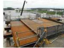
Platform installation completed (As announced on June 15, 2012)
