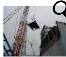
Lifting up the protection platform (As announced on June 15, 2012)
